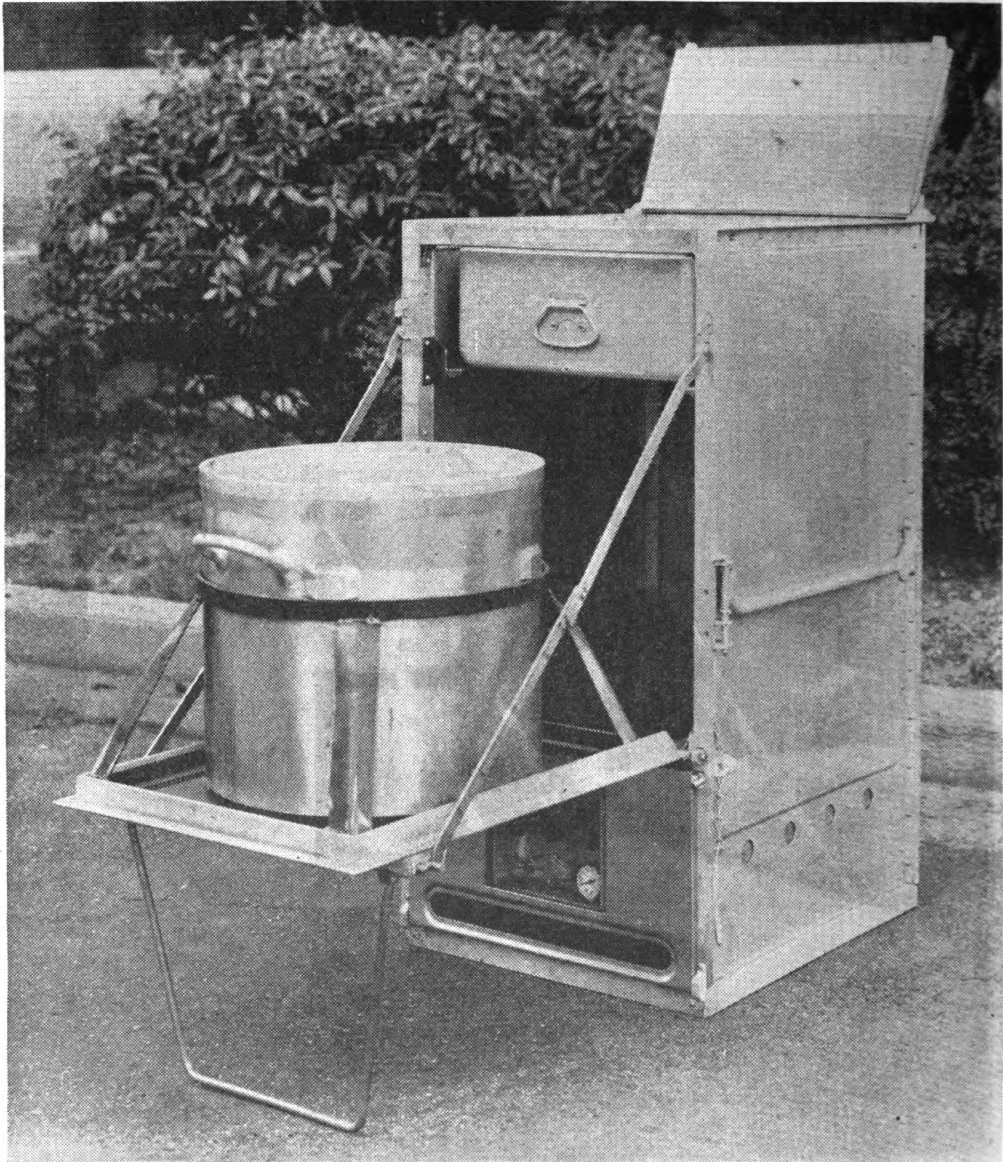
FIGURE 31.—One unit of the range with cooking vessels uncovered, and in position for serving food.
